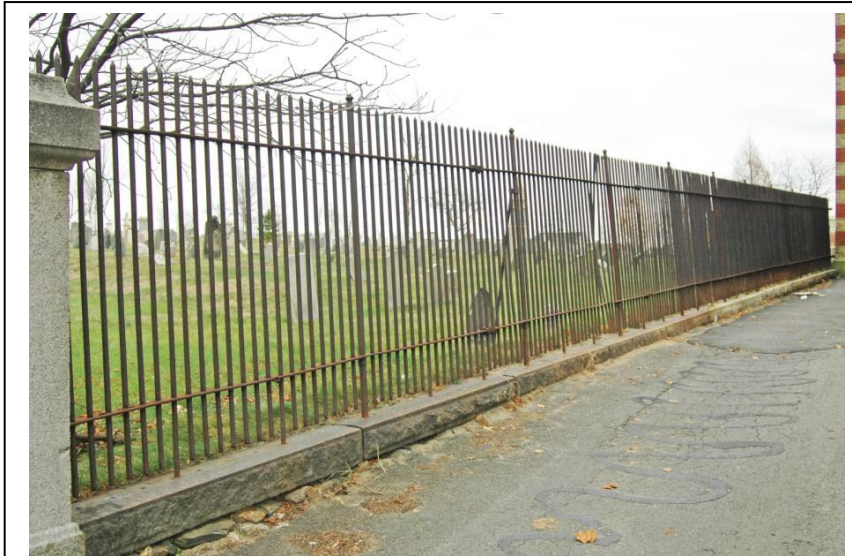
Figure 59. North School fence running from Congress to the North School alcove.
