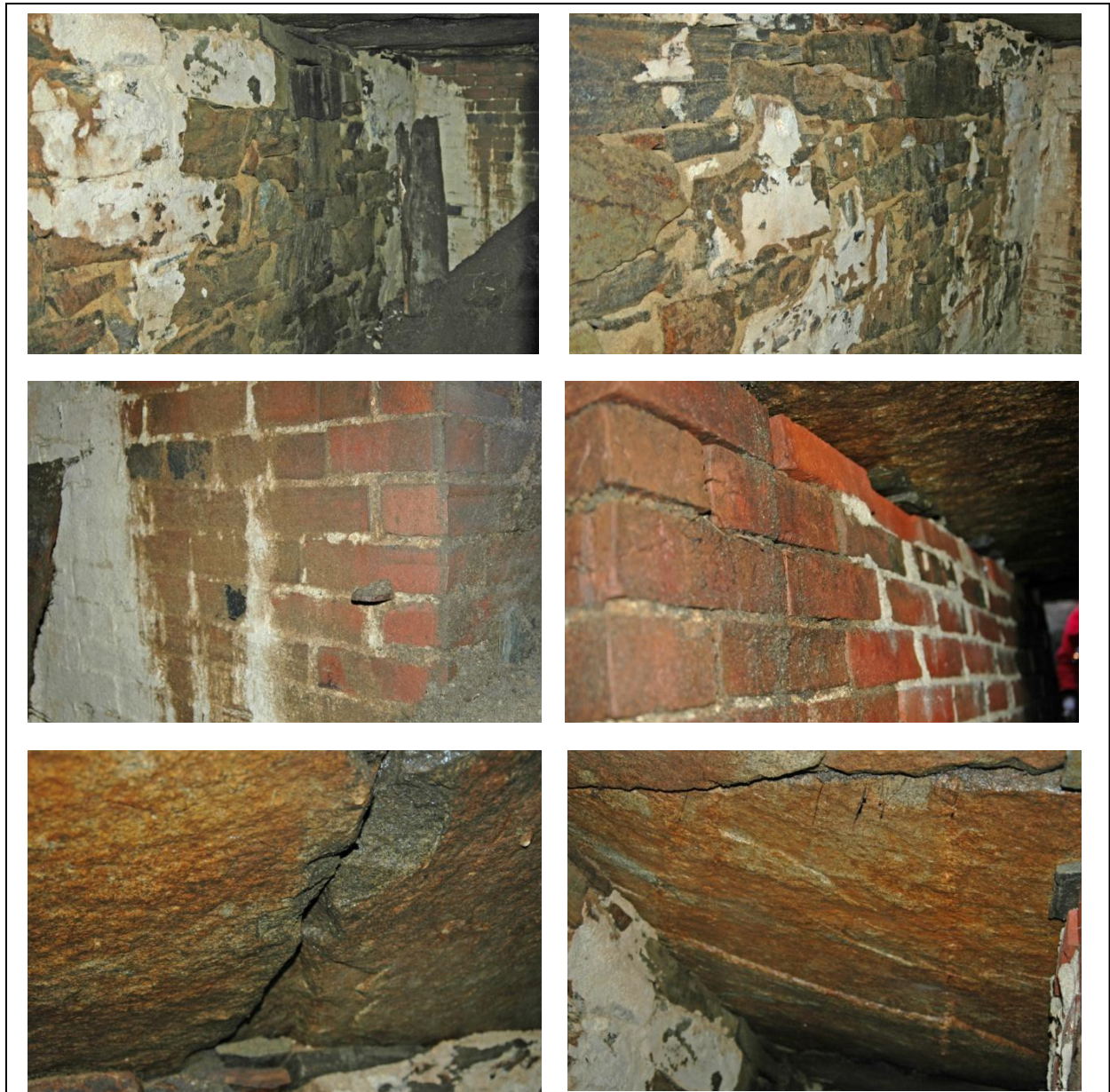
Figure 64. Dyer Tomb (A-22). Upper left photo is of the right (north) side wall looking toward the tomb opening (east). In the corner is part of the old plank covering. In the lower right of the photo is the soil spilling in from the tomb entrance. Upper right photo shows the left (south) side wall looking toward the back of the tomb (west). Middle left photo shows the brick wall north of the opening. Note the iron eye bolt. Middle right photo shows the added central wall, looking toward the tomb opening. Note repointed brick. This wall, unlike the tomb walls, has never been whitewashed. Lower left photo shows the wet ceiling of the tomb to the left (south) of the central wall (in the background). Lower right photo shows a crack in the ceiling.
