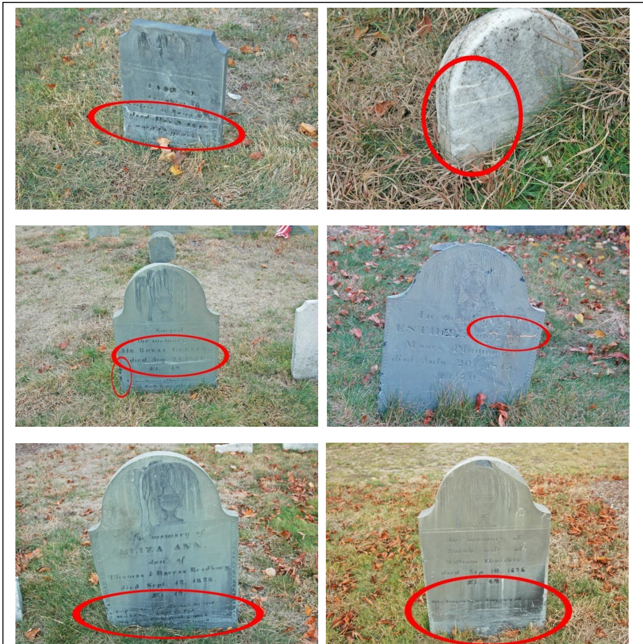
Figure 71. Examples of mower and trimmer damage to stones in Eastern Cemetery. Upper and middle photos show typical scrapes and damage caused by mowers. The photo on the middle right reveals paint transfer from the mower onto the stone itself. The photos in the bottom row show parallel striations on the stones caused by careless trimmer use with a line too heavy for cemetery work.
